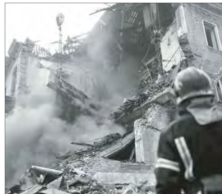
Ukrainian State Emergency Service firefighters clear the rubble at the building which was destroyed by a Russian attack in Kryvyi Rih, Ukraine, Friday, Dec. 16. Russian forces launched at least 60 missiles across Ukraine that day.
